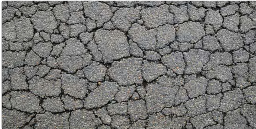
Fatigue cracking
