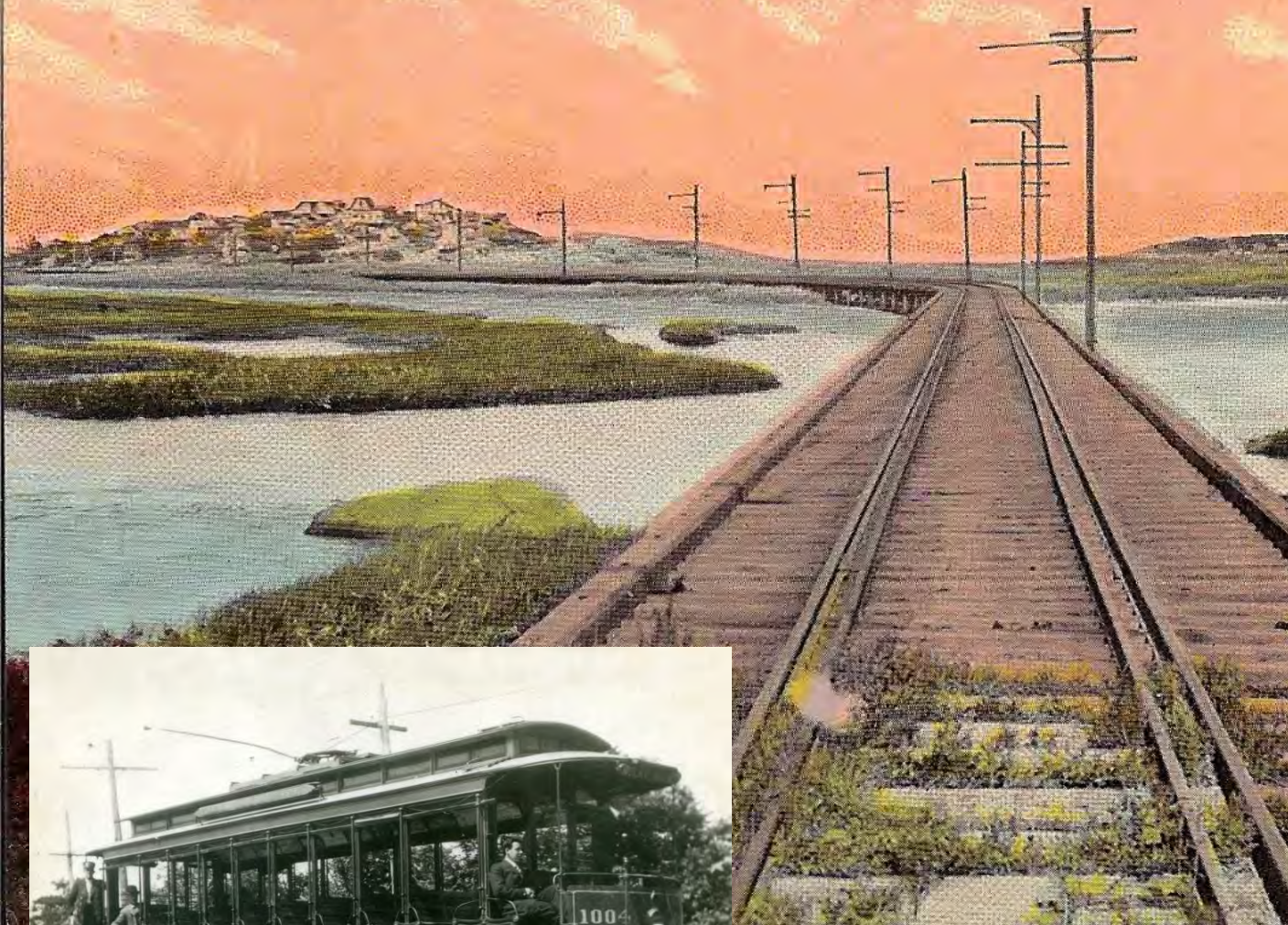
The Trestle across Little Good Harbor Beach, Bass Rocks, Gloucester, Mass.
