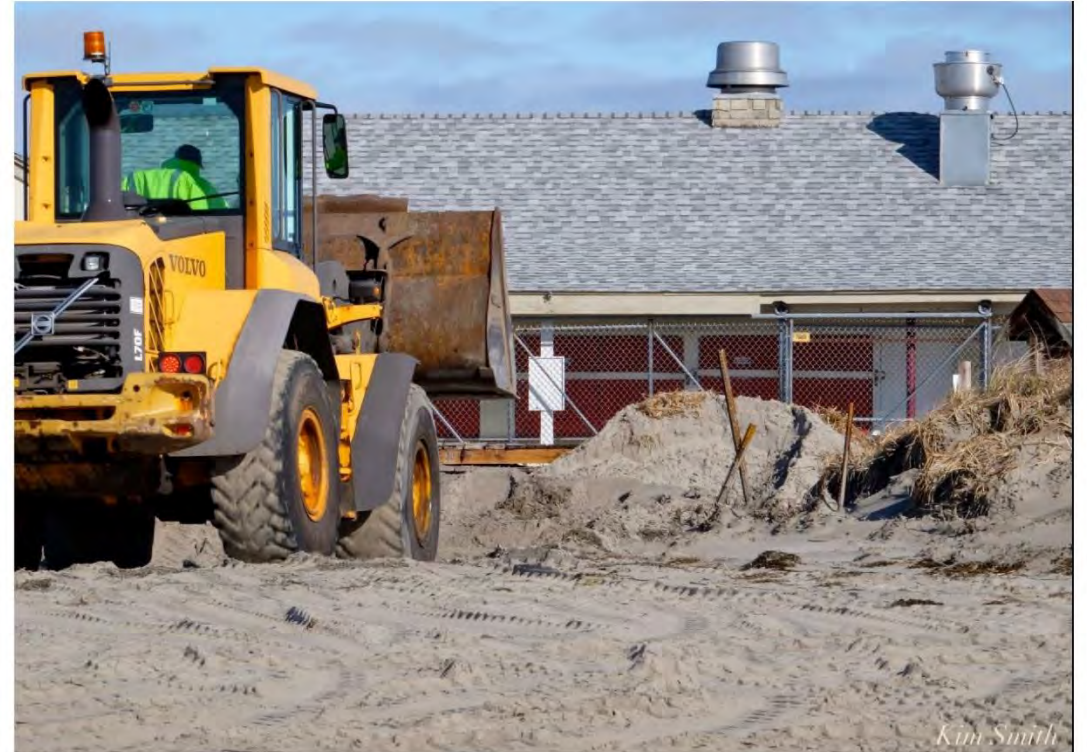
Kim Smith. Good Harbor Beach Storm Damage. 2018. Good Morning Gloucester.
